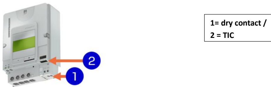
Figure 1: TIC and dry contact interfaces
